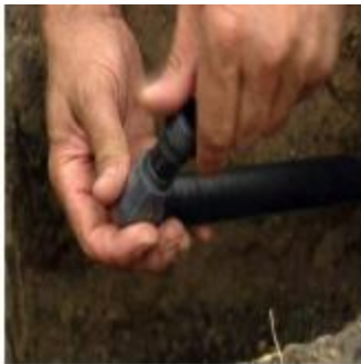
Run the PVC pipe
