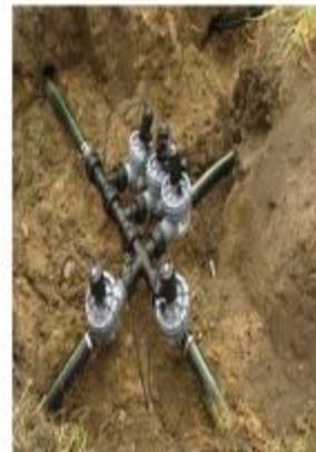
Install the Valve Manifold
