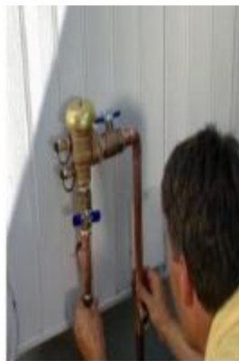
Access the Water Line
