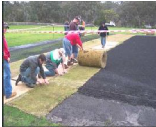
Laying washed sod
