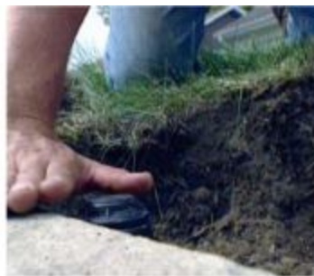
Install the Sprinkler Heads
