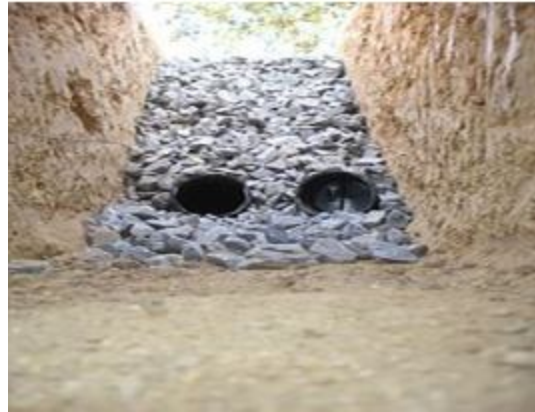
CROSS SECTION OF FRENCH DRAINAGE
